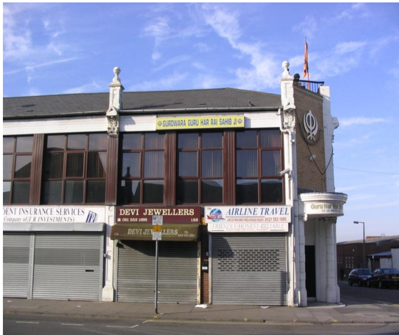
© Sandwell M. B. C. copyright. All rights reserved Figure 40 – Example of split level premises.
