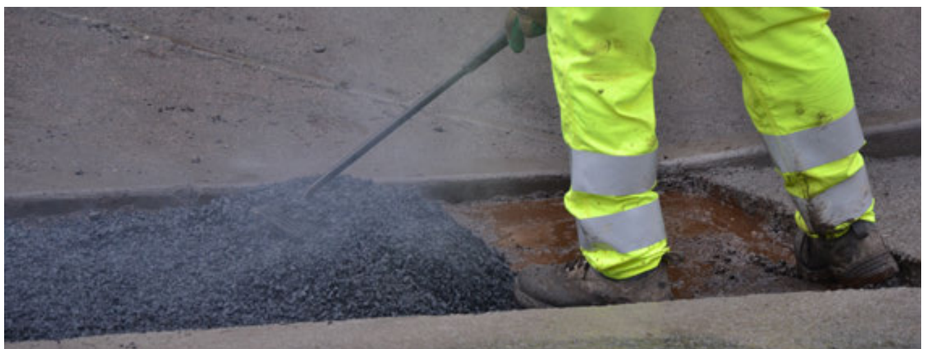
The hot Armaphalt material used as normal to complete the re-instatement.
